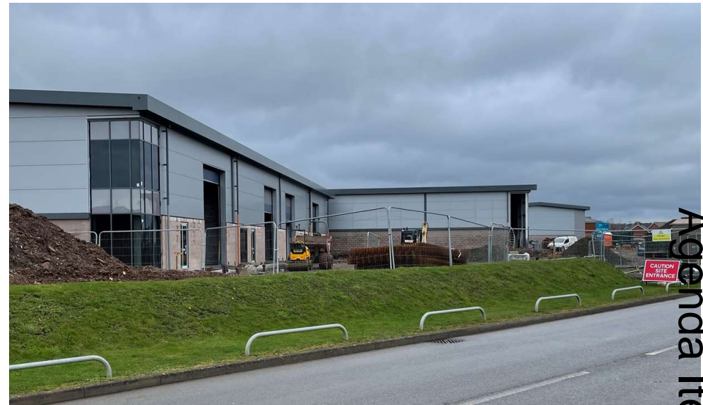
Construction opposite site
